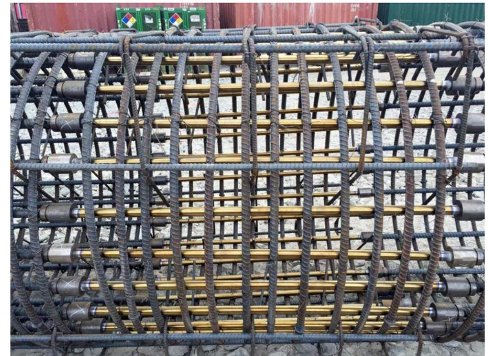
Bridge column rebar with SMA coupled to steel rebar.
