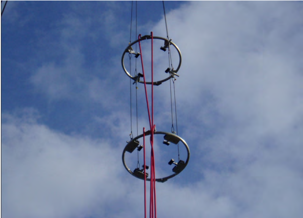
Figure 6: Photograph of the bubble curtain prior to deployment around the pile.
