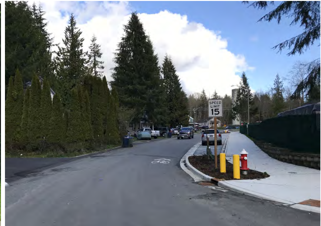
April 2023 Completed Walkway
