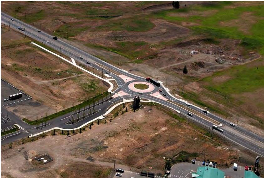
WSDOT EASTERN REGION FILE PHOTO. US2 SPOKANE TRIBE ROUNDABOUT. 2018, SPOKANE, WA.
