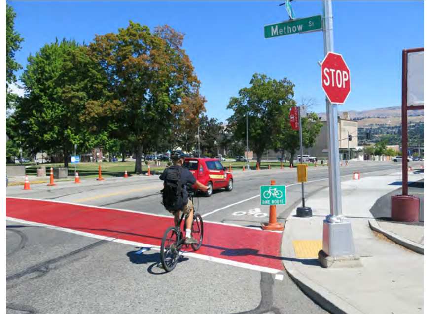
Wenatchee quick-build complete streets project. Source: Smart Growth America
